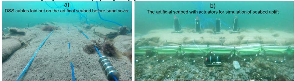
Fig. 3. (a) Three different configurations of DSS cables installed before covering with sand; (b) seafloor uplift actuators at the bottom, sand layer and pressure/inclination recording units placed on top during near-shore experiments outside Kiel
